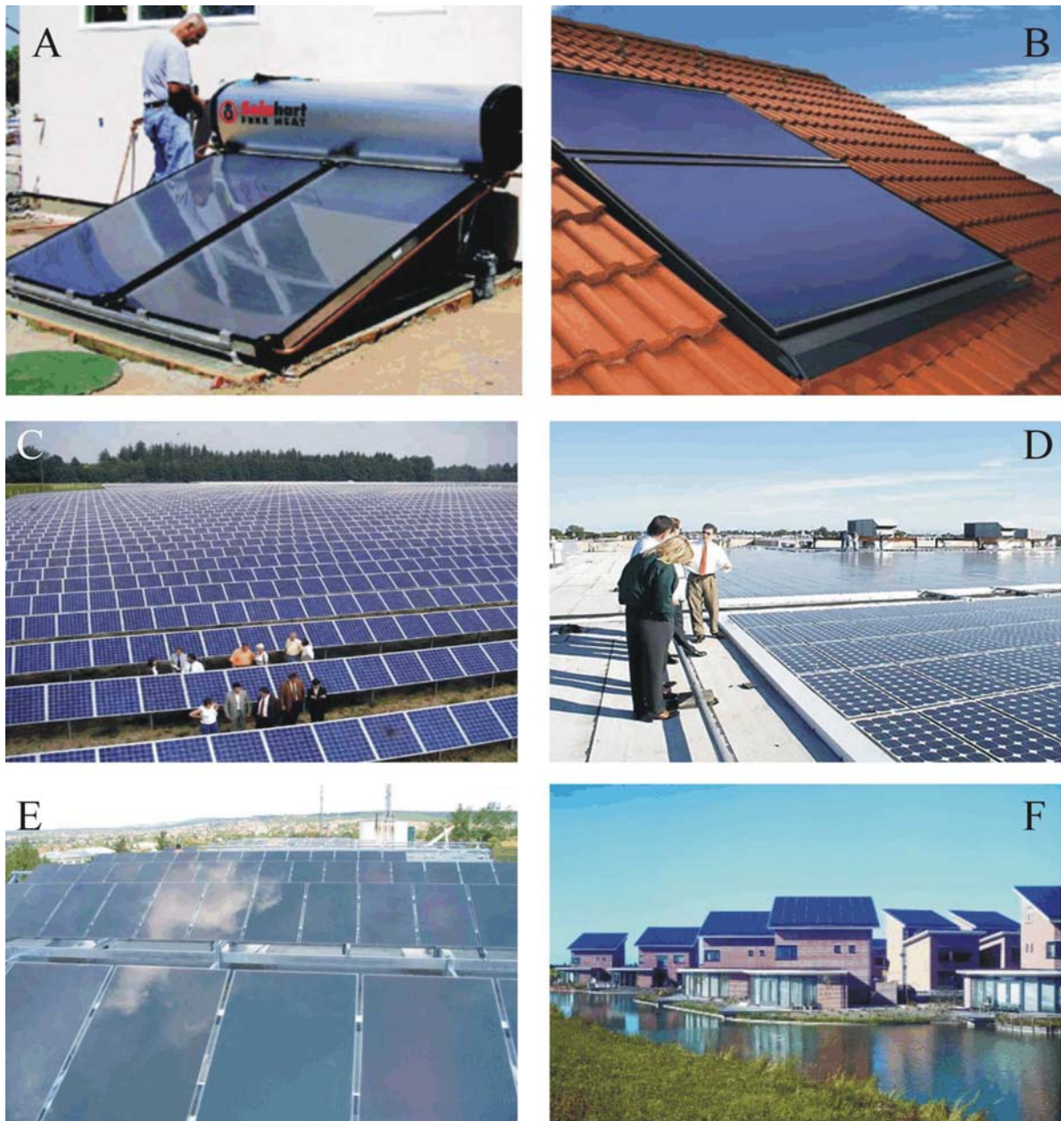
Figure 9.5. Solar panels, including solar collectors (SCs) and photovoltaic solar cells (PVSCs), are increasingly spreading in the world. (A) A passive, closed-circuit water heating system using a multi-flow shiny black solar collector panel providing high-efficiency absorption of solar radiation. The heated-up water is stored in black cylindrical tanks ( http://www.solahart.com ). (B) A SC on the roof of a house ( http://www.weishaupt.de ). (C) A German solar electricity plant with thousands of PVSCs ( http://www.phoenixsolar.com ). (D) Horizontal PVSCs on a rooftop in Farmingdale, Long Island, NY, USA ( http://www.power-technology.com/projects/long_island ). (E) PVSCs on the rooftop of a building of the Szent István University in Gödöllő, Hungary (photo by G. Kriska). (F) PVSCs on the roofs of family houses in the Japanese solar town, Kiyomino ( http://www.iea-pvps-task10.org ).
